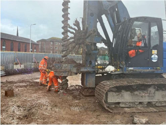
Figure 4-3: Piling Rig on working platform.
