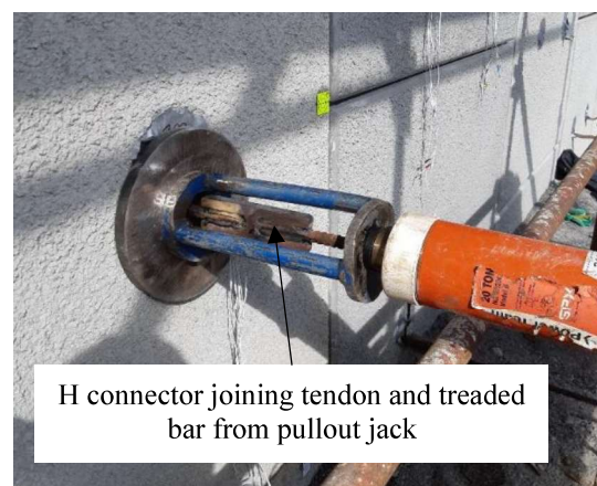
Figure 9. Connection between jack and anchor tendon during a test
